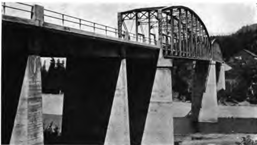
The Scotia bridge across Eel River on the State Highway. Humboldt County helped pay for this bridge.
